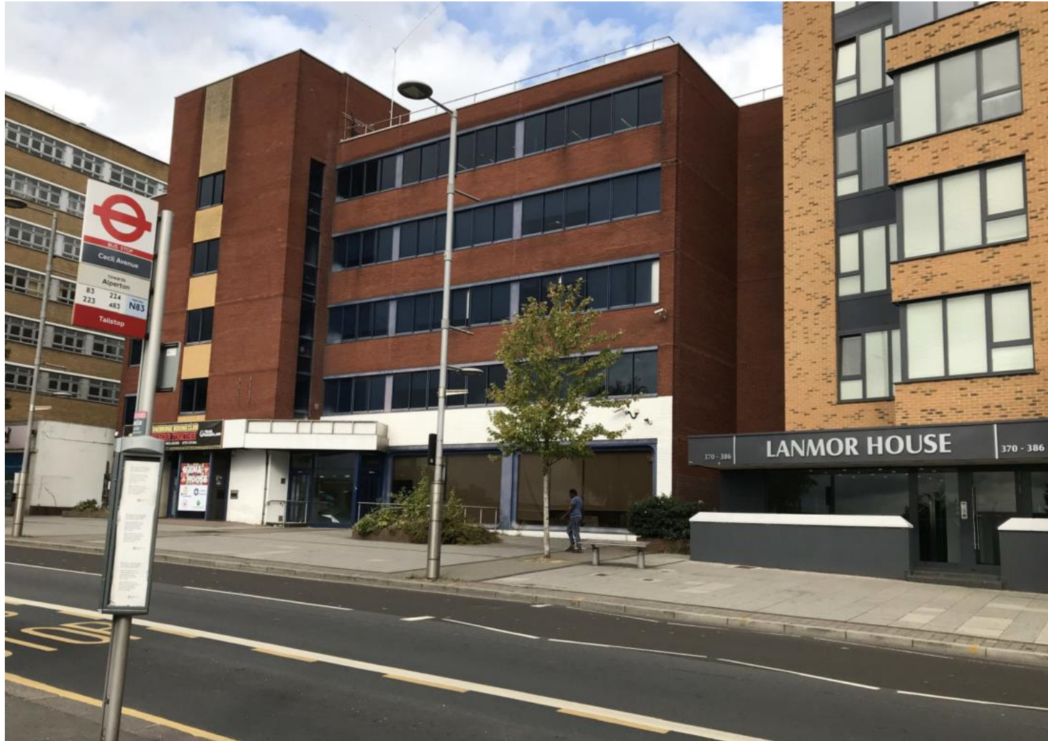
Photo 2: view of site from southeast
