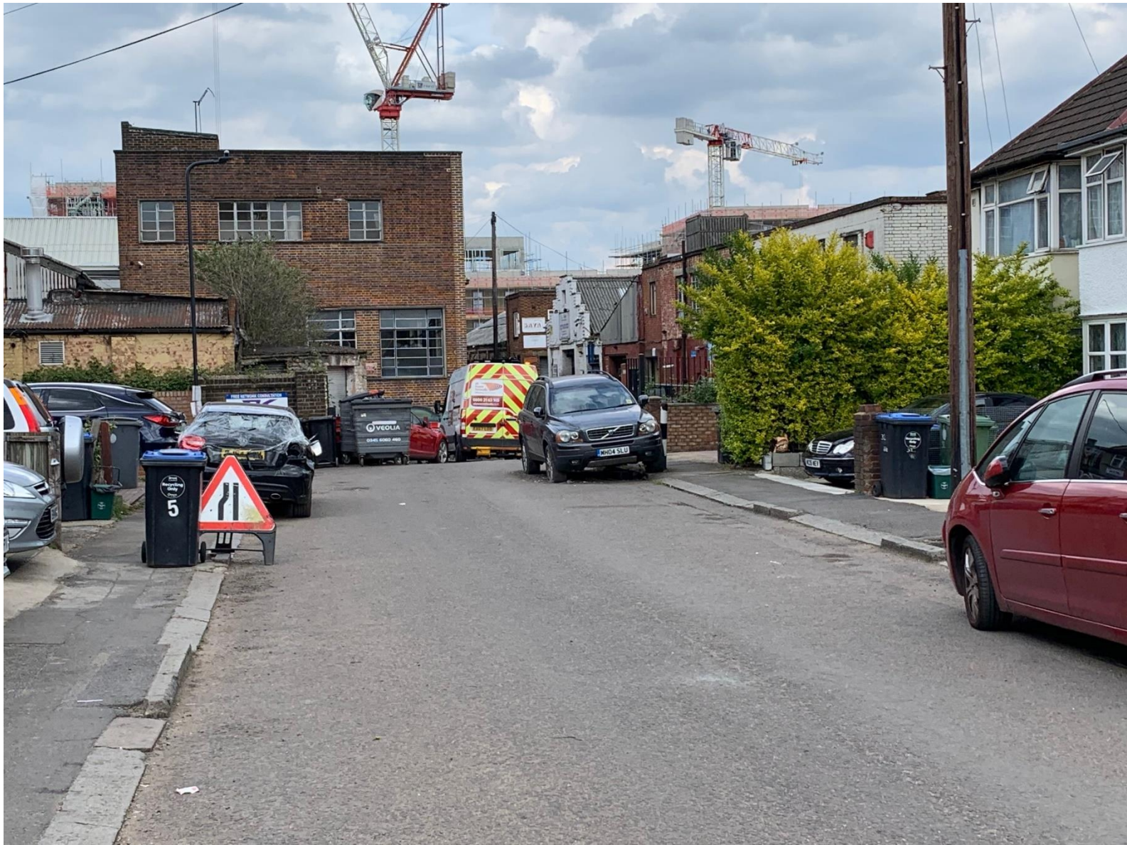
Photo 14: View of south western entrance to site from Woodside End
