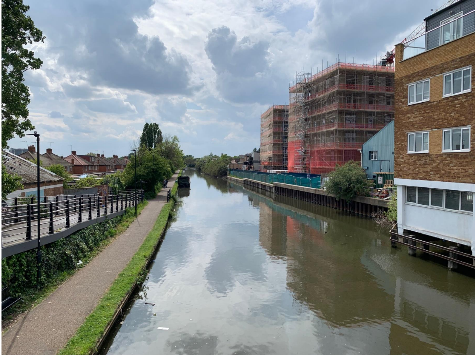
Photo 6: View from Liberty Centre towards Abbey Wharf and Abbey Manufacturing Estate beyond
