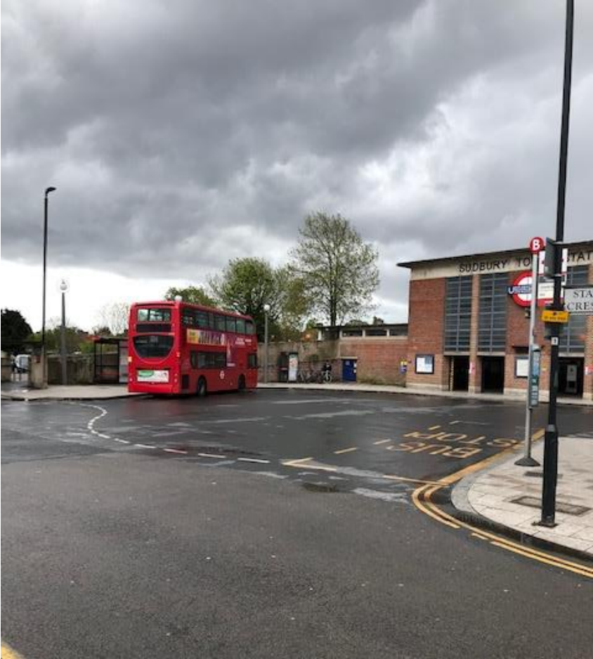
Photo 2: Front forecourt showing bus and taxi stand on Station Approach
